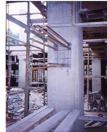
Connecting Beam to Column
